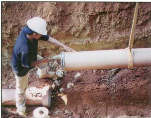
Applying Joint Compound
